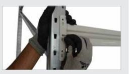
2 Click the remaining beams into place and attach the locking pins
